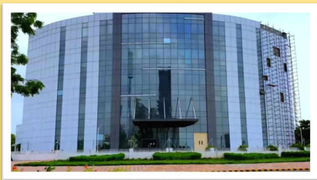
Tata Communications Tier IV Data Centre, GIFT City, Gandhinagar, Gujarat, India
