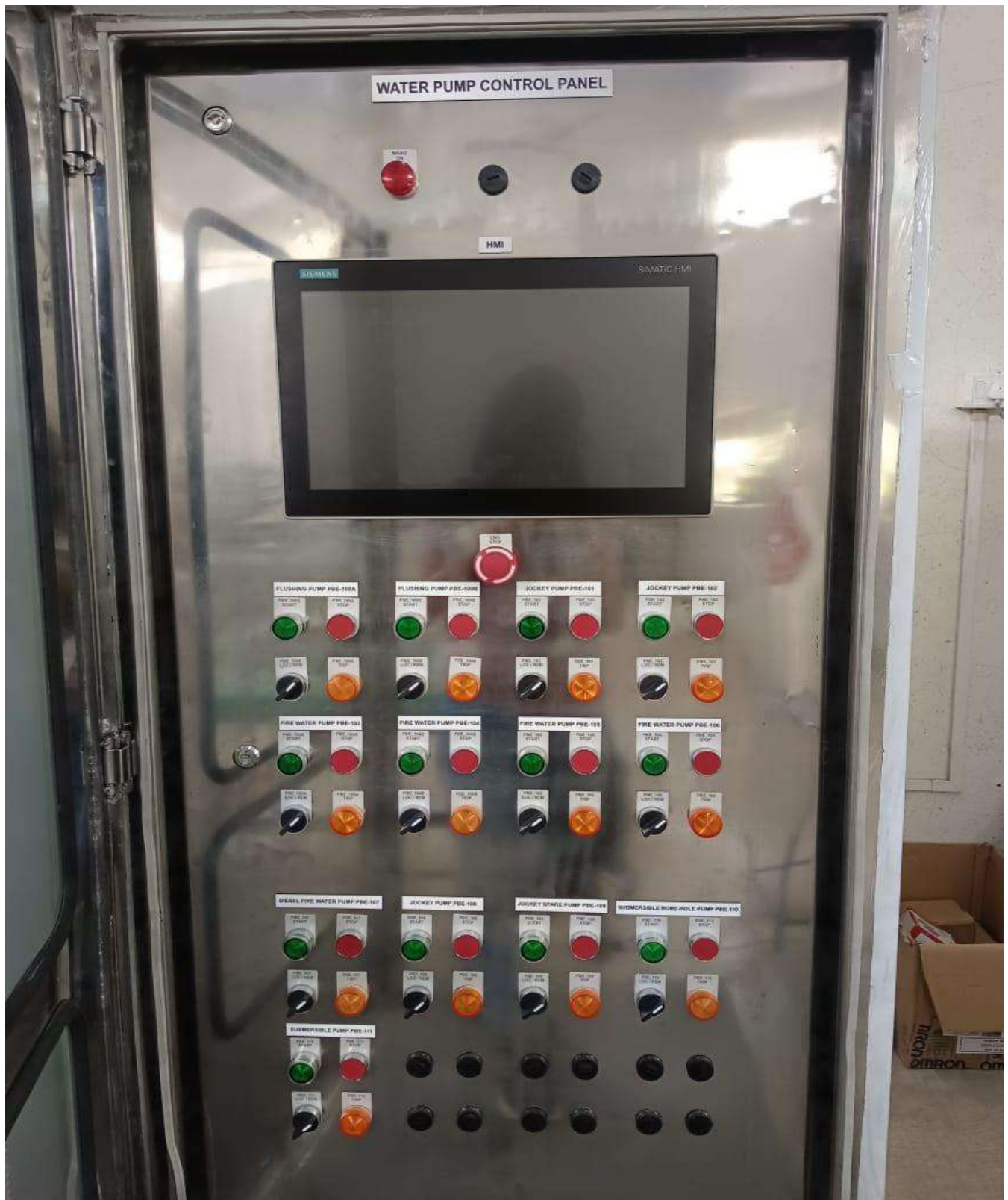
Figure Final water pump Control Panel
