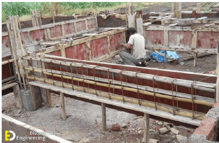
Fig. bamboo reinforcement
