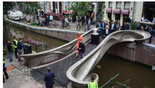
World's first 3D-printed steel bridge opens to public in Amsterdam Courtesy:The Hindu
