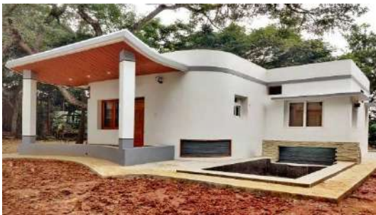
Indias first 3D printed House Built by IIT Madras startup Tvasta Courtesy: Times of India
