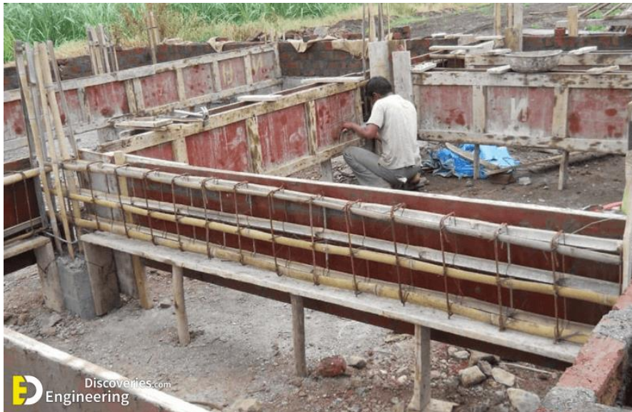
Fig. bamboo reinforcement
