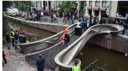
World's first 3D-printed steel bridge opens to public in Amsterdam Courtesy: The Hindu
