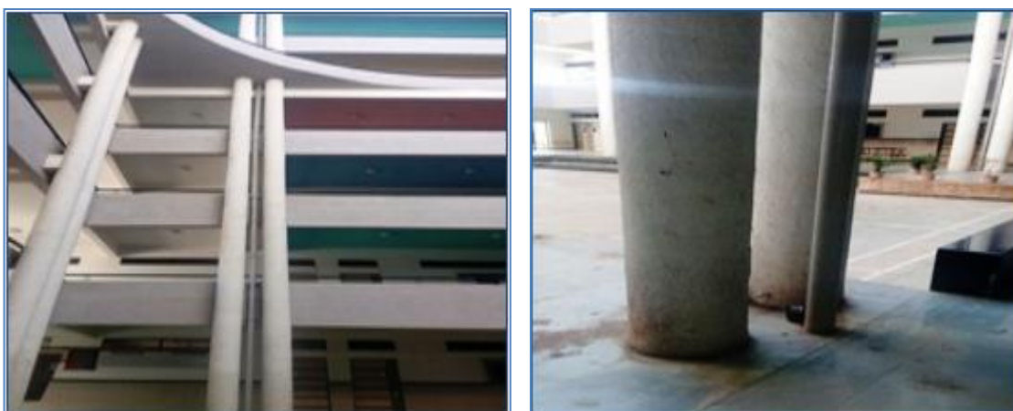
Fig. 7.1.2 (B): Water harvesting at academic building-C.
